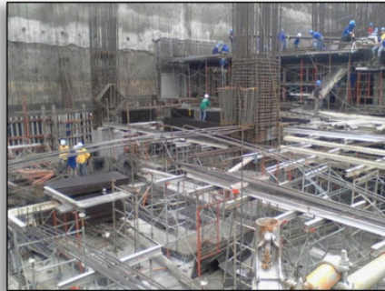
Formworks Installation, Uptown Mall, BGC
