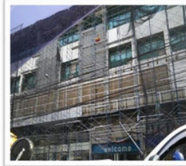
Scaffolding Installation, Newtown, Makati
