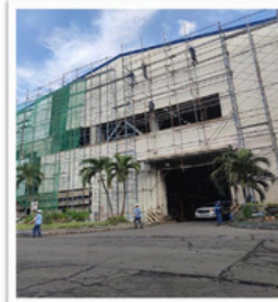
Scaffolding Installation, Carcar, Cebu
