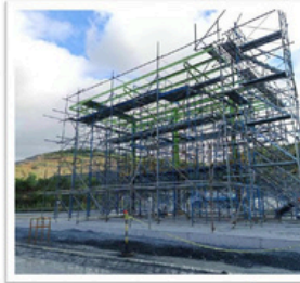
Scaffolding Installation, Angono, Rizal
