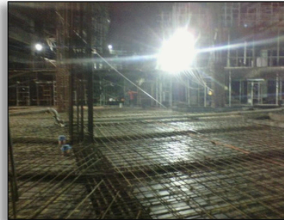
Rebar Installation, Uptown Mall, BGC
