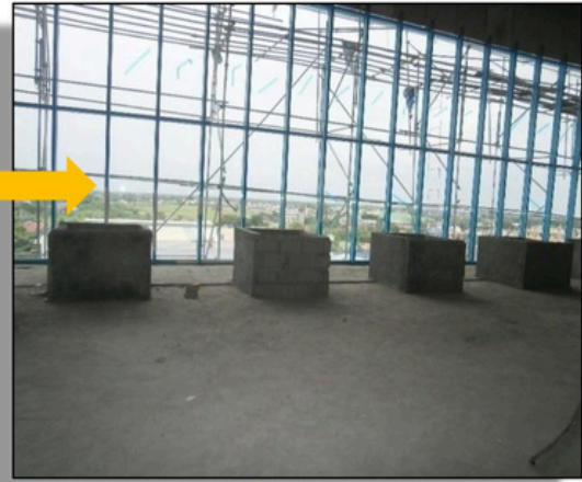
Installation of Fins, SM Cabanatuan, Nueva Ecija
