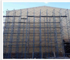
Scaffolding Installation, Calaca, Batangas
