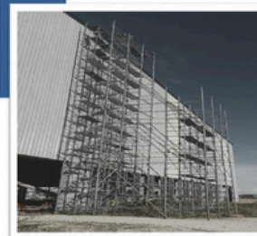
Scaffolding Installation, Compostela Cebu
