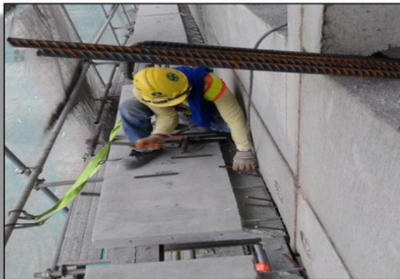
AC Ledge Installation, Amaia, Pasig City
