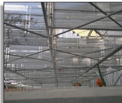
Scaffolding Installation Mama Sita's, Pasig City
