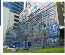
Scaffolding Installation for ASEAN ROK Mural Painting.
