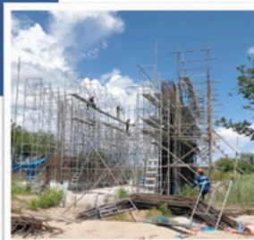
Scaffolding Installation, Floridablanca, Pampanga
