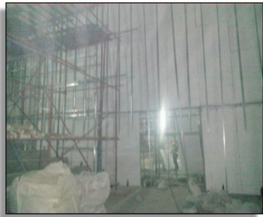
Dry Wall Installation, SM Cabanatuan, Nueva Ecija
