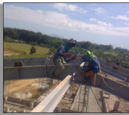
Warehouse Construction, Batangas City
