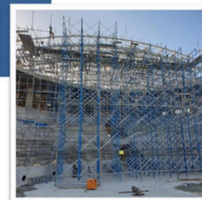
Scaffolding Supply, Candon, Ilocos Sur
