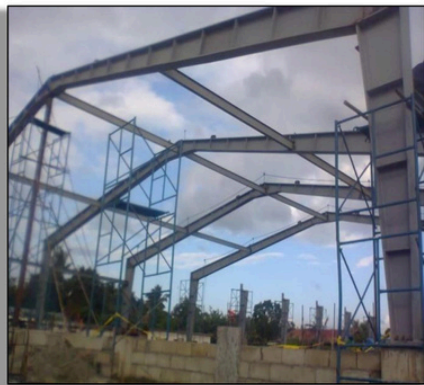
Warehouse Construction, Batangas City
