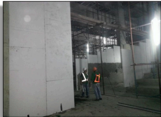
EPS Wall Installation, Seda Vertis North
