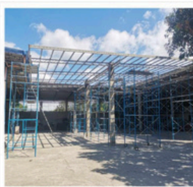
Scaffolding Installation, Kimja Motorpool Binangonan
