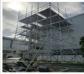
Scaffolding Installation, Sta. Rosa, Laguna
